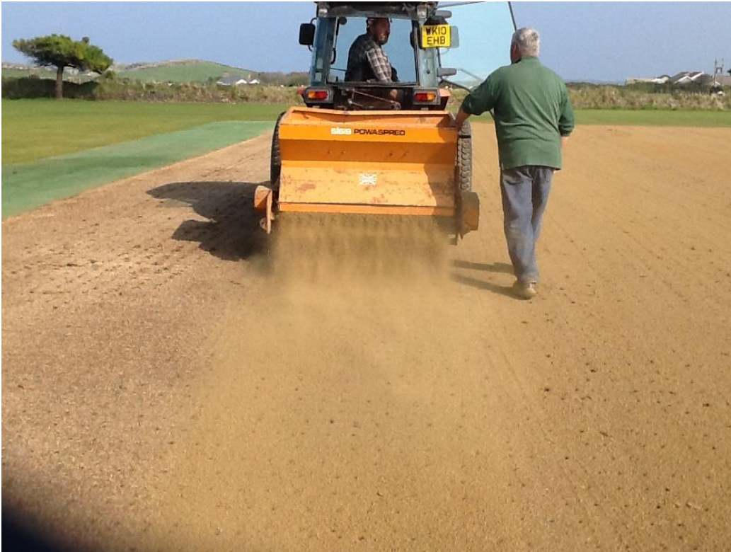
Application of Loam
